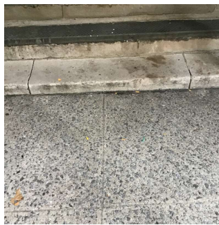
Facade A Door 3
