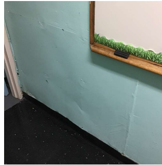
Corridor near Room 200
