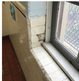
Corridor near Room 304
