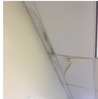
Roof 4 - Room 417 (Roof 4 - Library, Rooms 420, Roof 5 - Room 401, Roof 6 - Room 402 similar)
