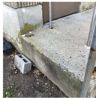
Facade A No violations recorded.
