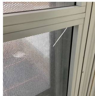
Facade D - Room 116
