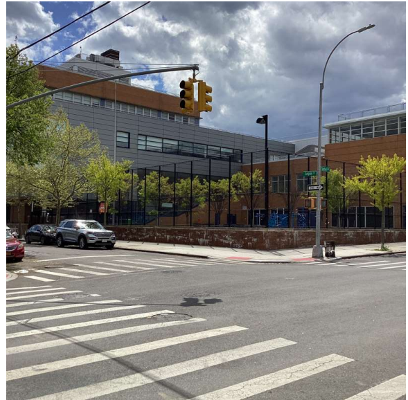
Corner of Sutter Avenue and Legion Street - Southwest View
