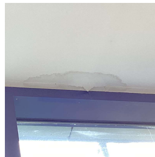
Facade A - Corridor near Room 223
