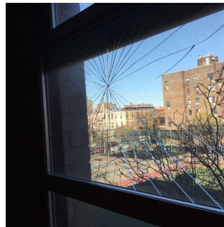
Facade J - 3rd Floor Corridor (Facade J - 2nd Floor Corridor, Facade K - Room 107 similar)
