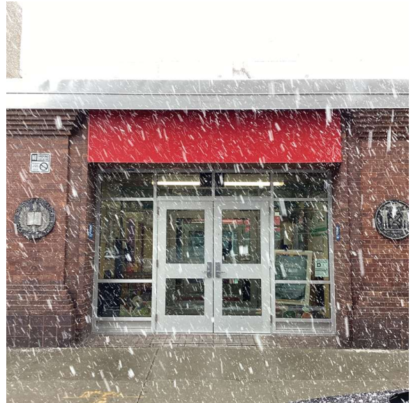
Facade A - Keap Street
