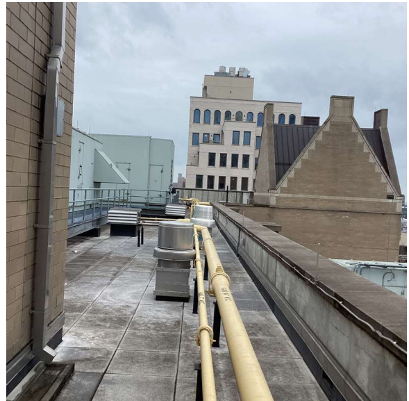
Roof 1 - Southwest View
