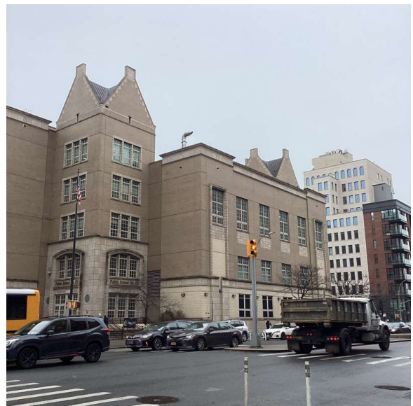
Corner of 4th Avenue and Baltic Street - Southeast View
