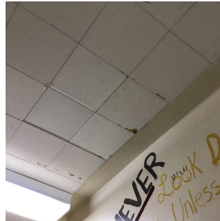
Corridor near Room 308
