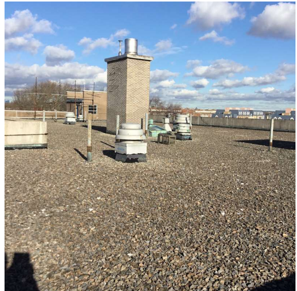
Roof 1 - North View
