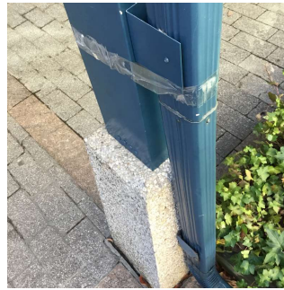
Main Entrance Canopy No violations recorded.
