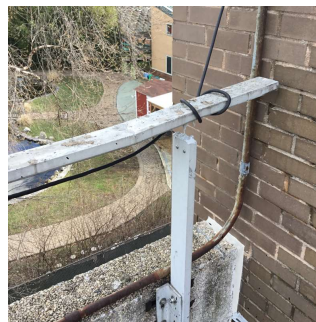
Roof 2 No violations recorded.
