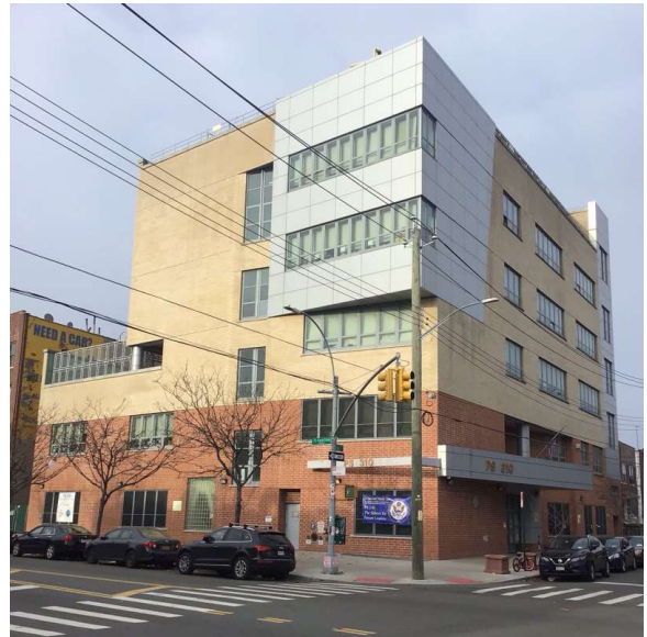
Corner of 62nd Street and Fort Hamilton Parkway - West View
