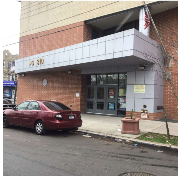
Facade A - 62nd Street
