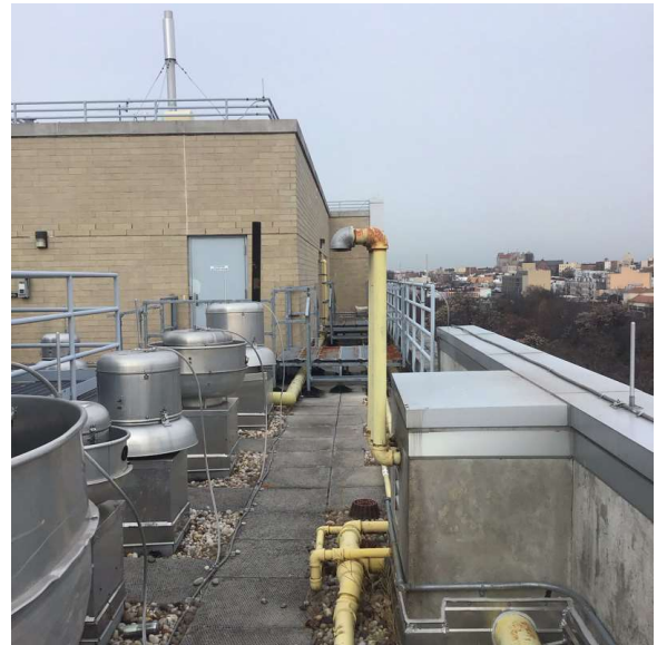
Roof 1 - Northwest View
