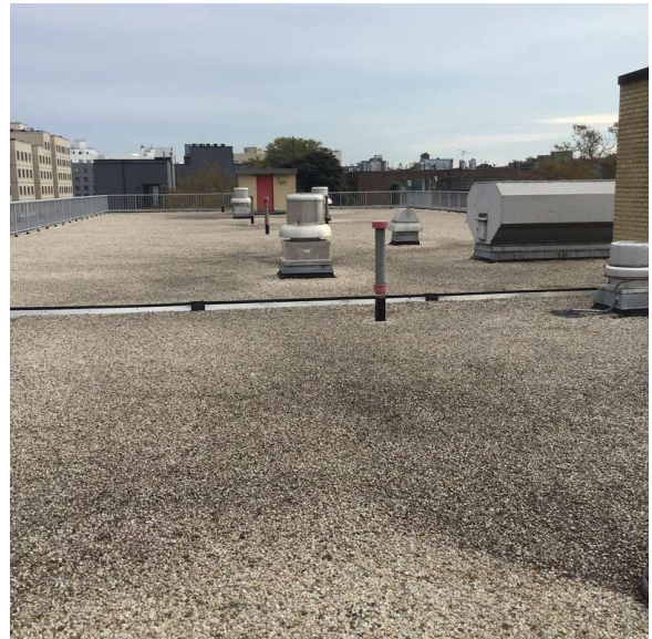
Roof 1 - West view
