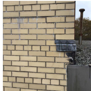
Roof 5 - East View
