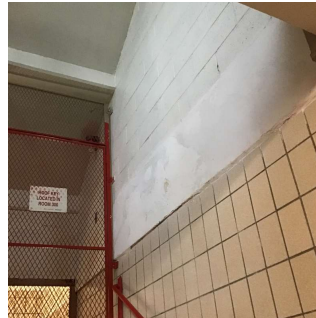
Roof 1 BH2 - Stair G/3
