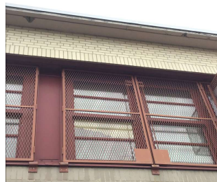
Roof 1 - Facade E
