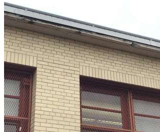
Roof 1 - Facade E
