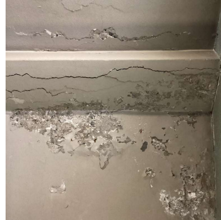
Stair D Bulkhead
