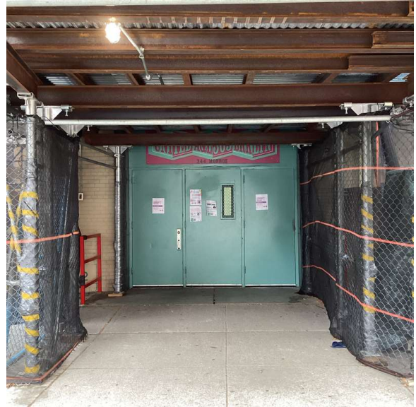
Facade A - Monroe Street
