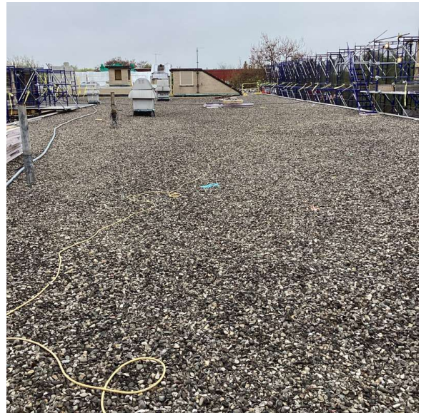
Roof 1 - Northeast View
