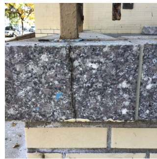
Facade A near Exit 2 No violations recorded.
