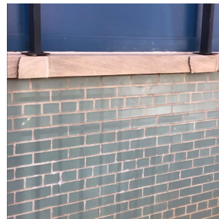
Facade A - West View
