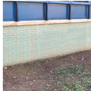
Facade A - West View
