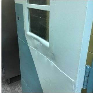
Entrance from Cafeteria
