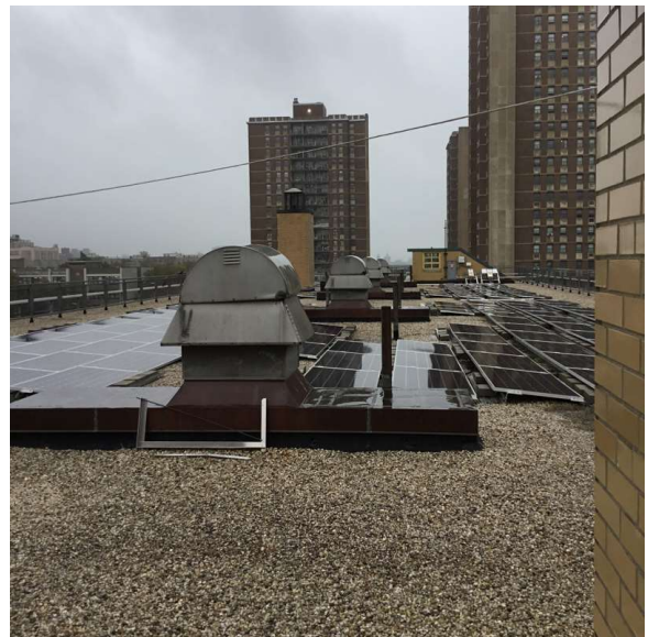
Roof 1 - East View
