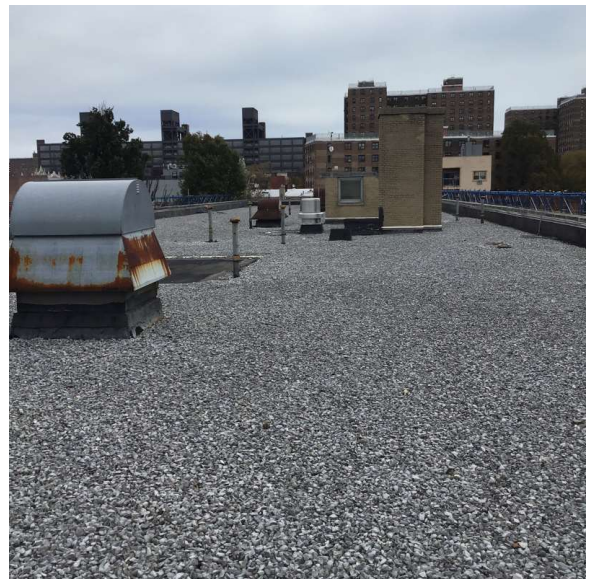
Roof 1 - East view
