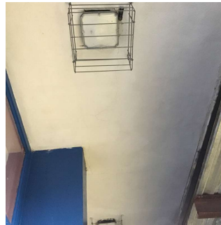
Main Entrance Canopy No violations recorded.
