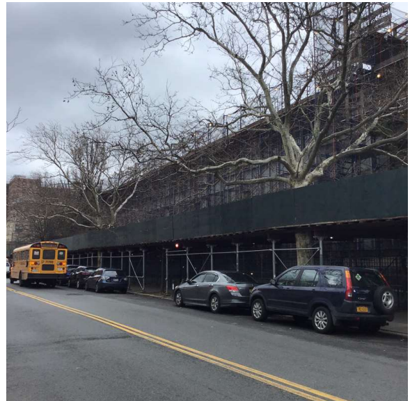
Park Avenue - Southwest view
