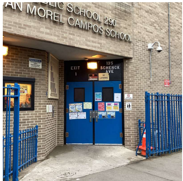
Facade A - Schenck Avenue
