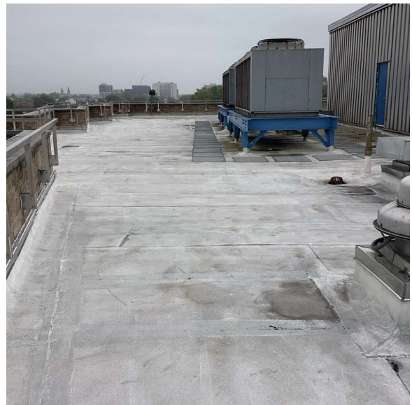
Roof 1 - West View
