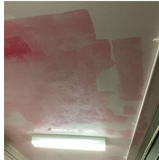
Corridor near Room 319
