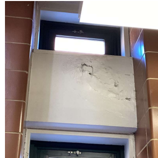
Facade B - Stair B/3, Facade D - Stairs D/3 (Shown)
