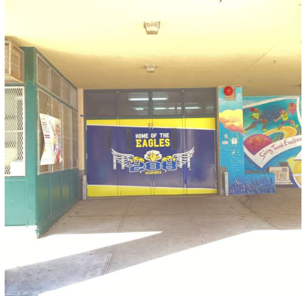
Facade A - West 25th Street
