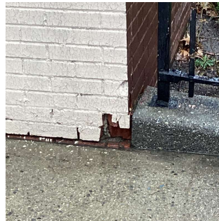
Corner of Facade H and Facade J
