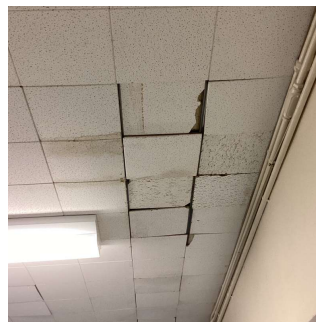
Corridor near Cafeteria
