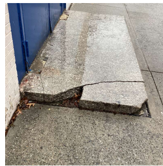
Facade B - Exit 3 No violations recorded.
