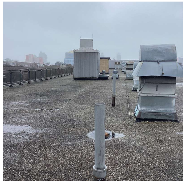
Roof 1 - Northwest View
