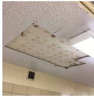
Corridor near Cafeteria
