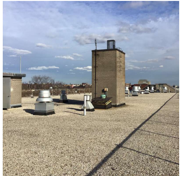
Roof 1 - South View
