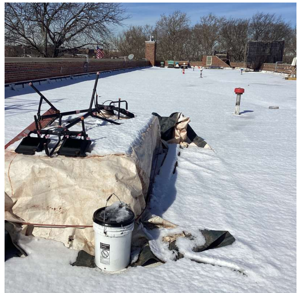
Roof 1 - Northwest View
