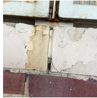
Facade F - Near Exit 12
