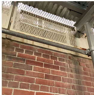
Facade H - Near Exit 11 No violations recorded.
