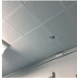
Corridor near Room 258
