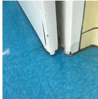
Corridor near Room 252
