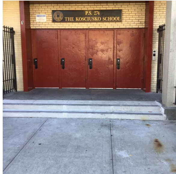
Facade A - Bushwick Avenue
