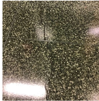
Stair D/1 Vestibule
