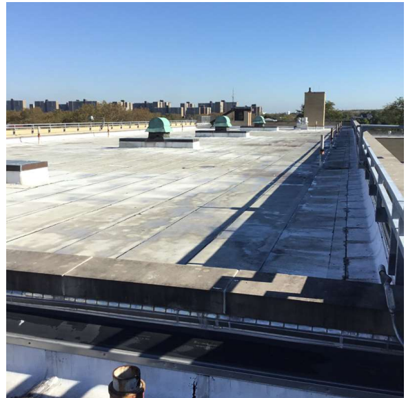
Roof 1 - Northeast View
