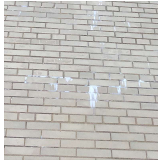
Facade at Roof 2
