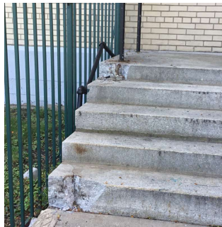
Facade B - Exit 3
