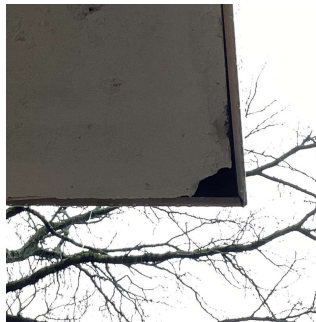
Facade A No violations recorded.
