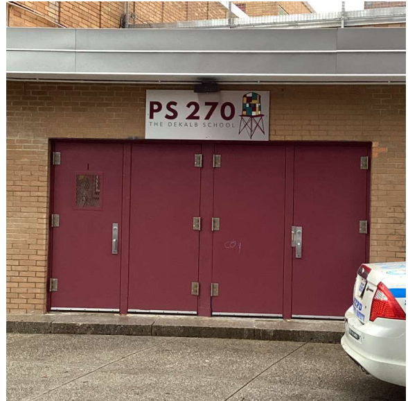
Facade A - East View
