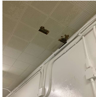
Corridor near room 317
