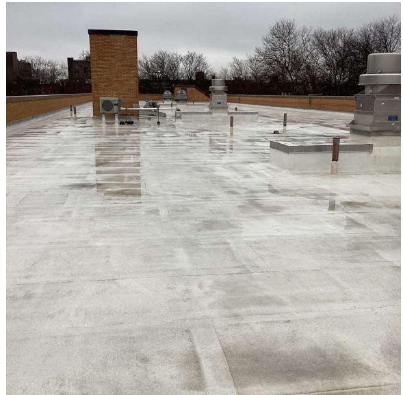
Roof 1 - South View
