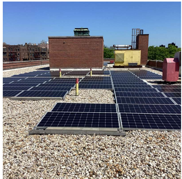
Roof 1 - North View
