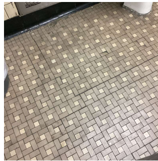
Men Toilet Room - 1st Floor
