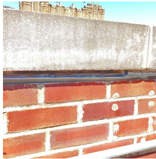
Roof 1 - Facade A
