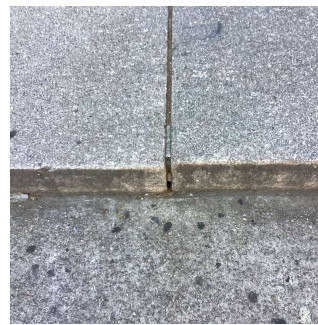
Facade A - Main Entrance No violations recorded.
