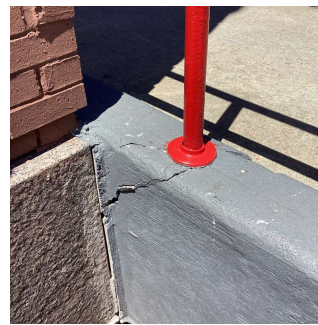
Facade L - HC Ramp No violations recorded.
