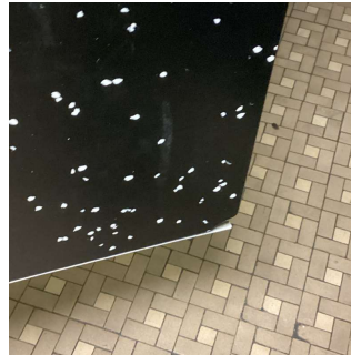
Women Toilet Room - 1st Floor
