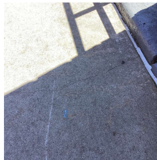
Facade L - HC Ramp
