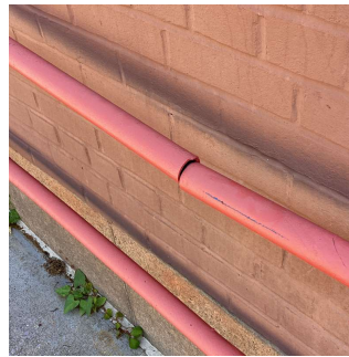
Facade A - HC Ramp
