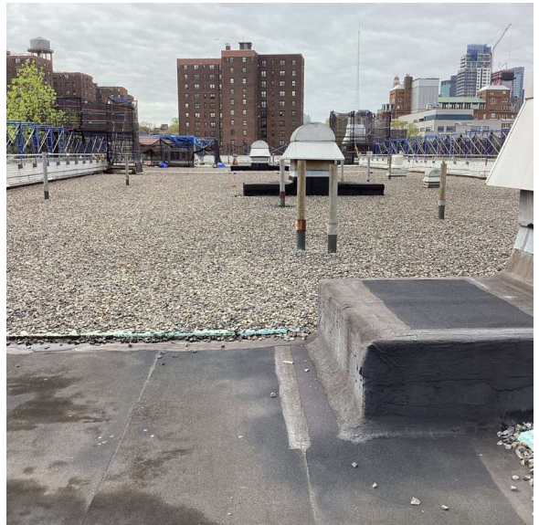
Roof 1 - South View
