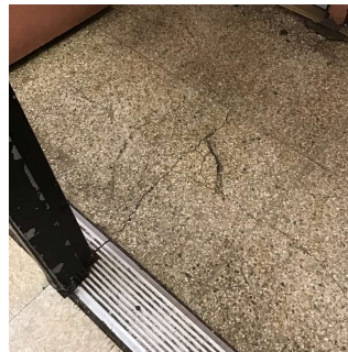
Stair B/1 Vestibule
