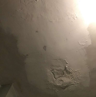
Roof 1 - Closet in Room 330 (shown), Room 312
