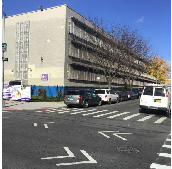
Corner of Chester Street and Blake Avenue - Northwest View
