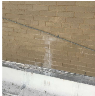
Roof 1 - Facade H
