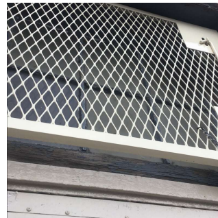
Facade F - Near Exit 9
