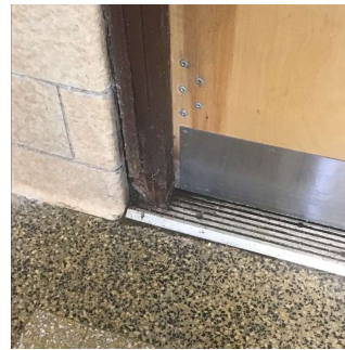
Facade A - Exit 4
