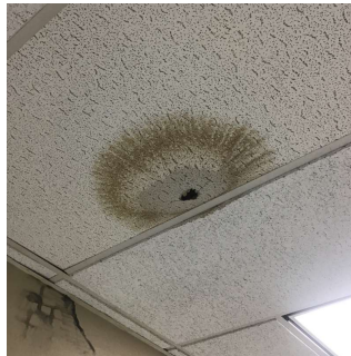
Roof 4 - Corridor near Room 432D shown, Roof 4 - Corridor near Room 437 similar
