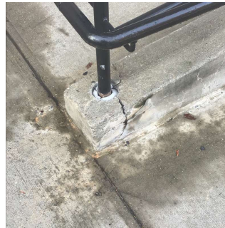
Facade A - HC Ramp
