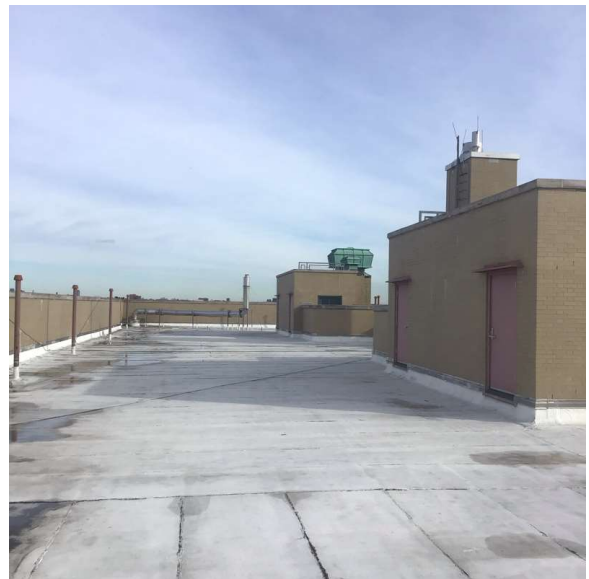
Roof 1 - Northeast View
