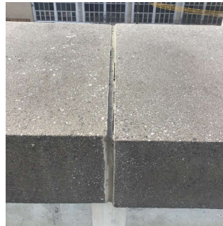
Roof 4 - Facade C No violations recorded.
