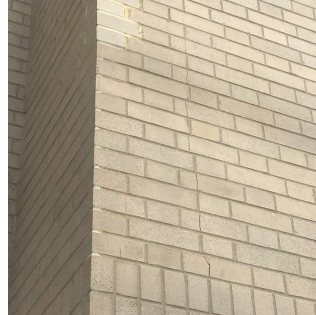
Facade G - Near Exit 8
