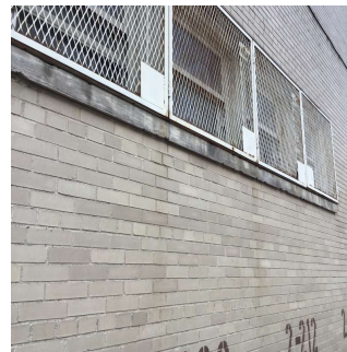
Facade C East View
