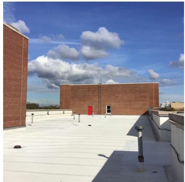
Roof 1 - Northwest view
