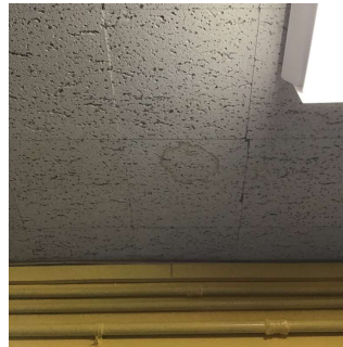
Corridor near Room 320
