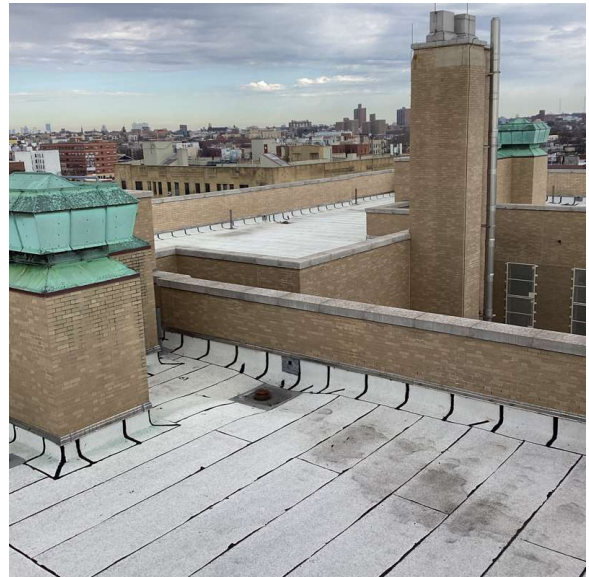
Roof 1 - North View
