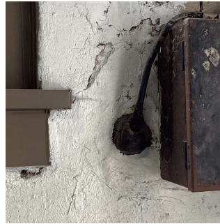
Basement Fan Area (Crawl Space under Auditorium similar)
