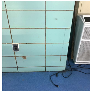
Near water fountain
