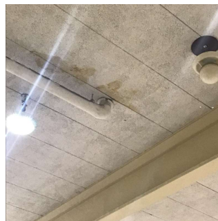
Roof 3 - Gymnasium, Roof 2 - Room 131 similar
