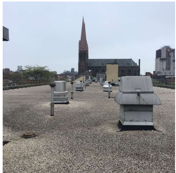
Roof 1 - Northeast View
