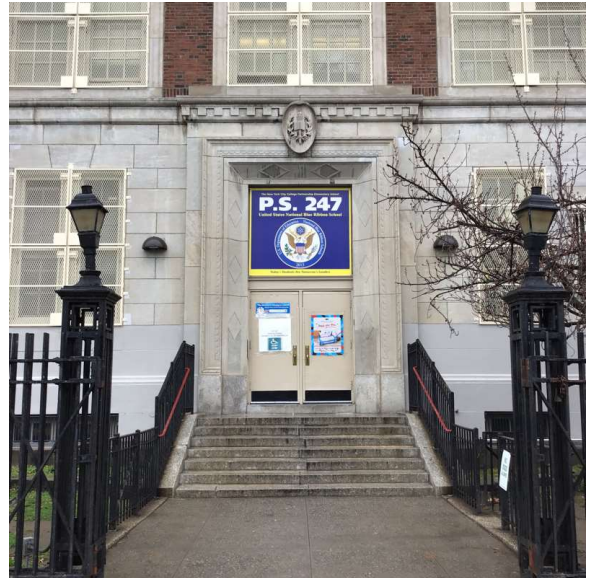
Facade A - 21st Avenue
