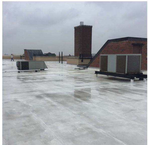
Roof 1 - West view
