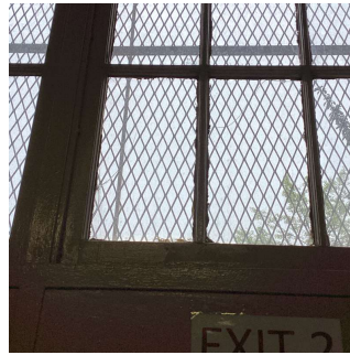
Facade A - Exit 2
