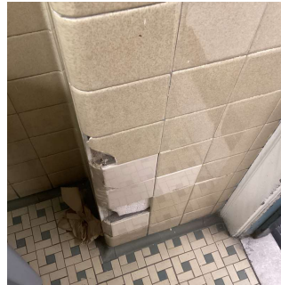
Staff Toilet Room - 3rd Floor
