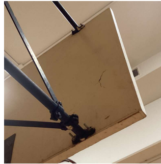
Near Stair H/4
