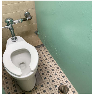
Staff Toilet Room - 3rd Floor
