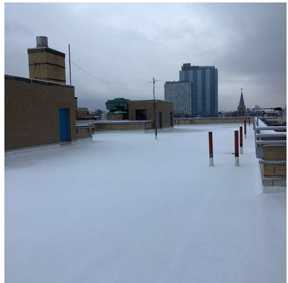
Roof 1 - Northwest View
