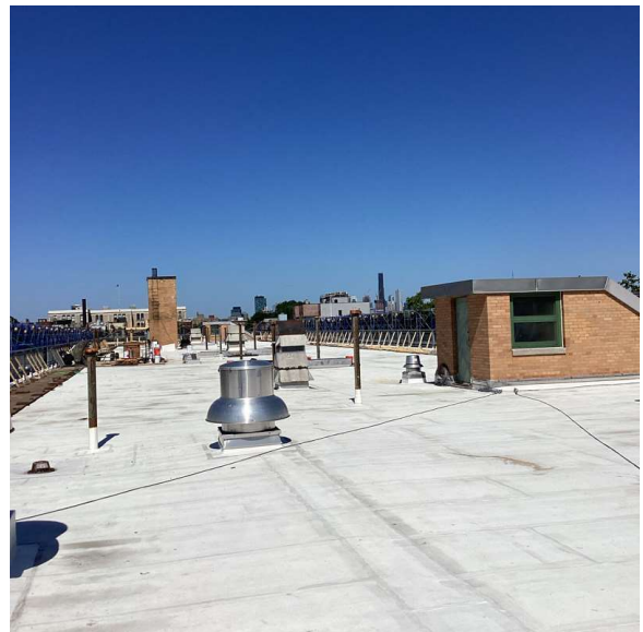
Roof 1 - West View
