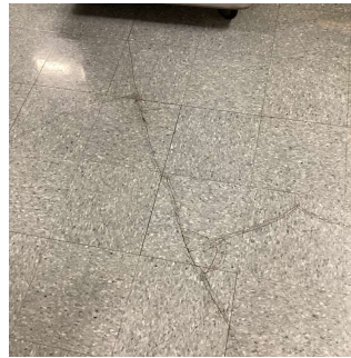
Near Kitchen Entrance No violations recorded.
