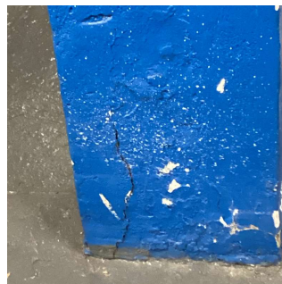
Boiler Room (Basement Storage Area, Oil Tank Room similar)
