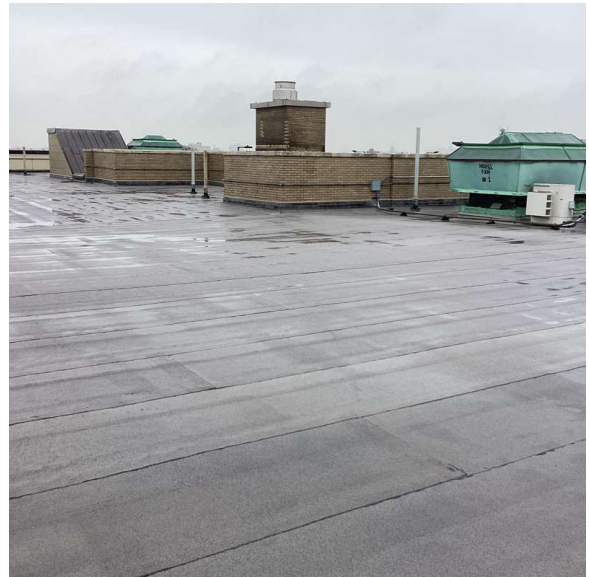
Roof 1 - North View
