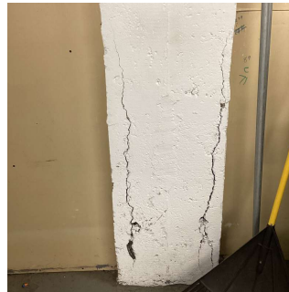
Basement Storage Room (Oil Tank Room, Boiler Room similar)
