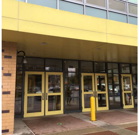
Facade A - Avenue P
