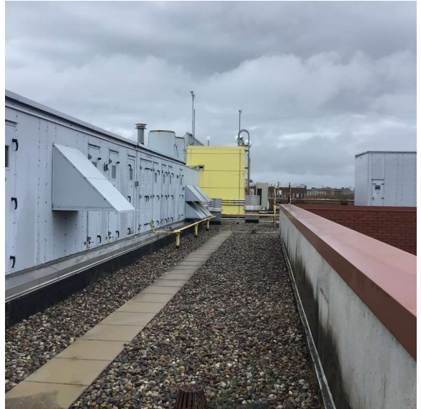
Roof 1 - North view
