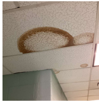
Corridor near room 305
