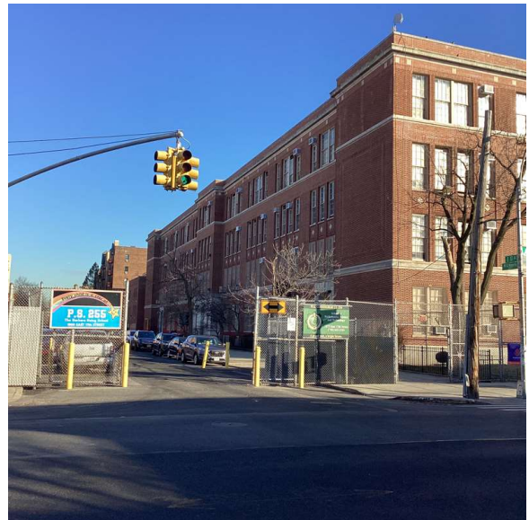
Corner of East 17th Street and Avenue S - Northeast View
