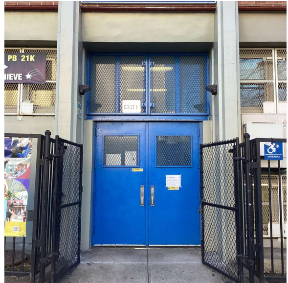
Facade A - 36th Street
