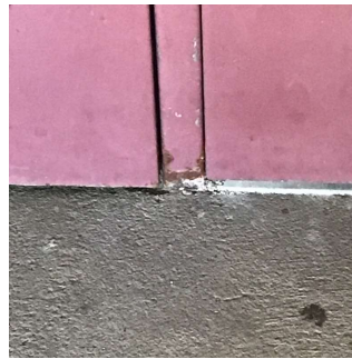
Facade C - Exit 6
