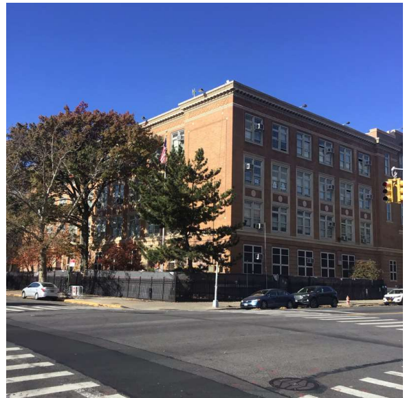
Corner of Albemarle Road and McDonald Avenue - Northwest View
