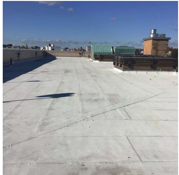
Roof 1 - West View
