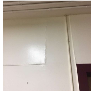
Corridor near Room 329
