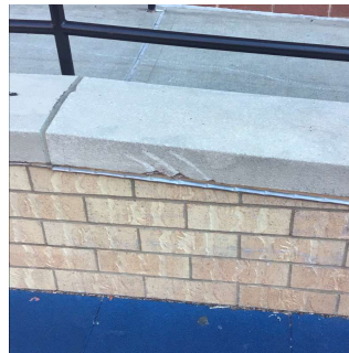
Facade C - Exit 2
