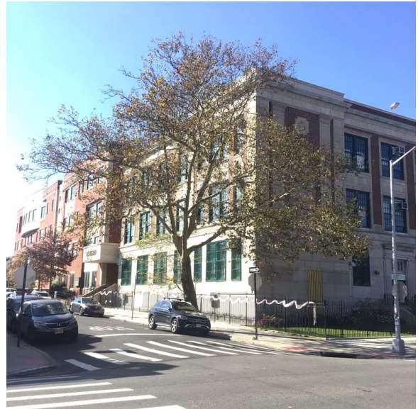
Corner of Benson Avenue and 14th Avenue - South View
