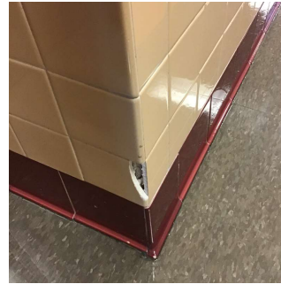
Corridor near Room 354
