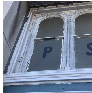
Facade H - Exit 9
