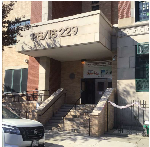
Facade A - Bay 7th Street
