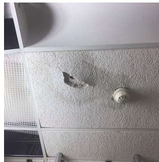
Roof 4 - Room 450 shown, Roof 3 - Room 449 similar
