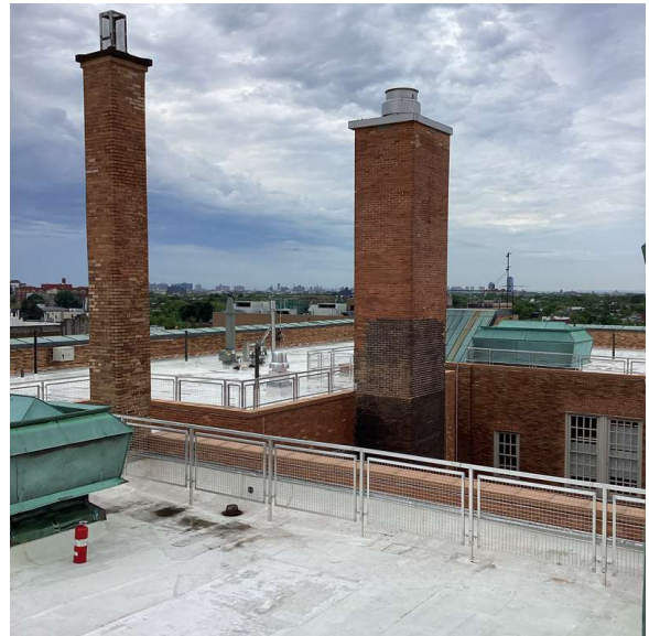
Roof 1 - Southeast View
