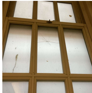
Facade D - Cafeteria Boy Toilet Room (Facade H - Auditorium similar throughout)
