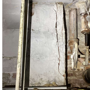
West Crawl Space (Basement Tile Storage Room similar)
