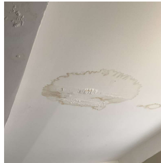
Roof 3 - Stairwell F/4+
