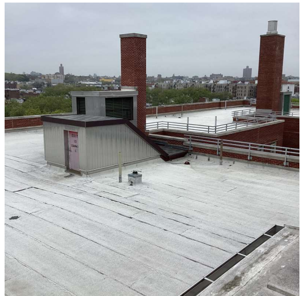
Roof 1 - North View
