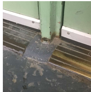
Facade D - Exit 5
