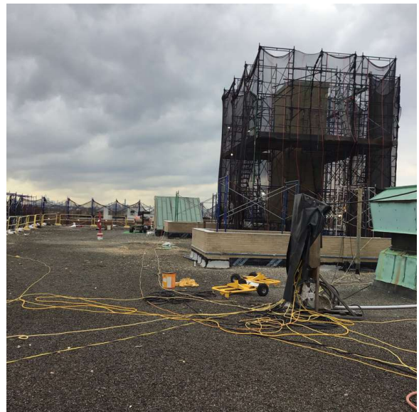
Roof 1 - North View
