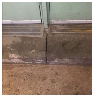
Facade C - Exit 3
