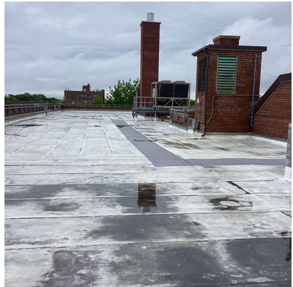
Roof 1 - West View
