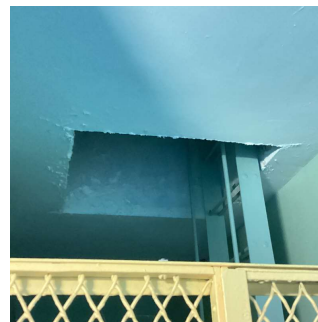
RH - Stair I (Non-instructional space)
