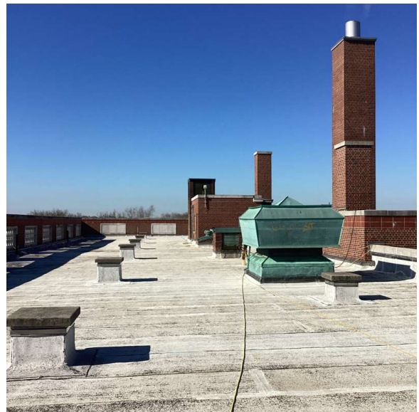
Roof 1 - Southwest View
