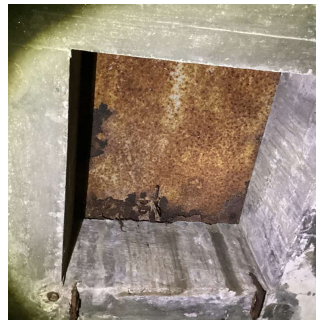
Ash Hoist Vault
