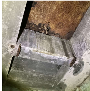
Ash Hoist Vault
