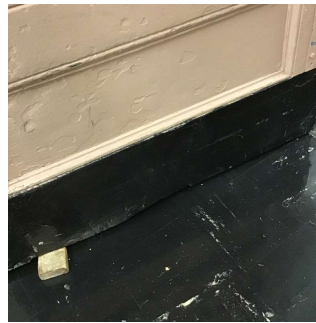
Corridor near Room 411
