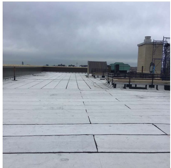
Roof 1 - Southeast View
