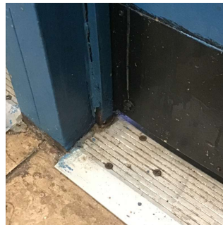
Facade C - Exit 10
