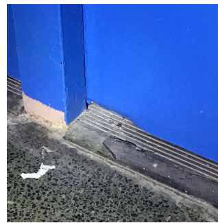
Facade H - Exit 6
