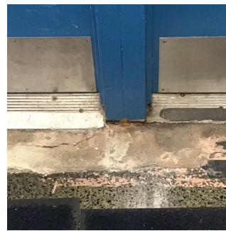
Facade A - Main Entrance No violations recorded.
