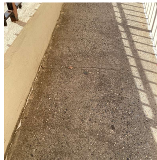
Facade H - HC Ramp
