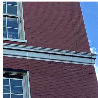
Facade B - Near Exit 2
