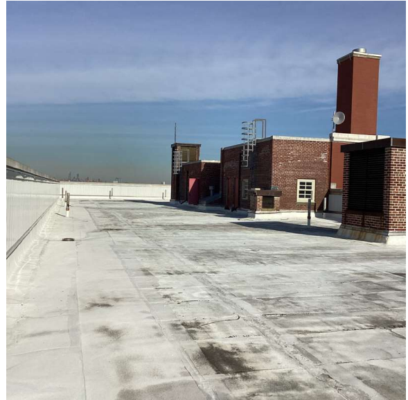
Roof 1 - Southeast View
