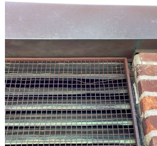
Roof 1 - Near BH1
