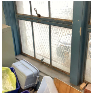
Facade E - Boiler Room
