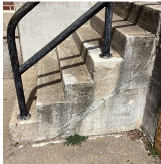
Facade E - Exit 10
