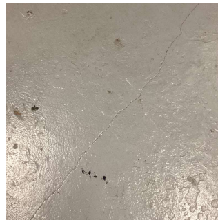
Boiler Room (Crawl Space similar)
