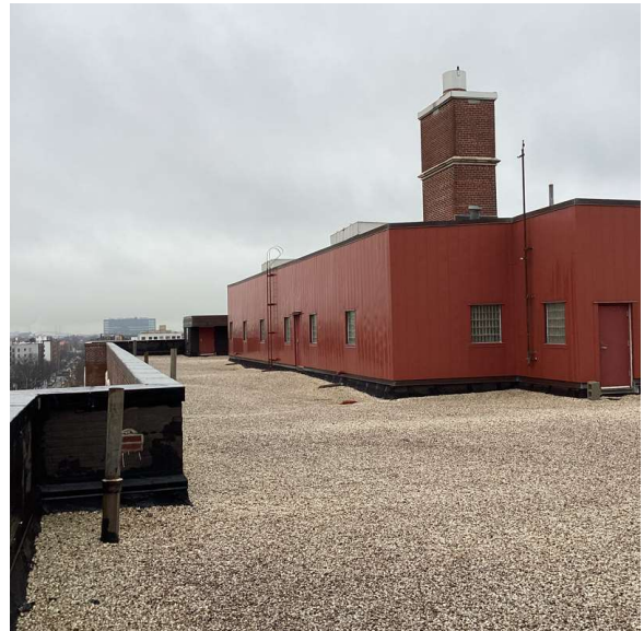
Roof 1 - Northwest View
