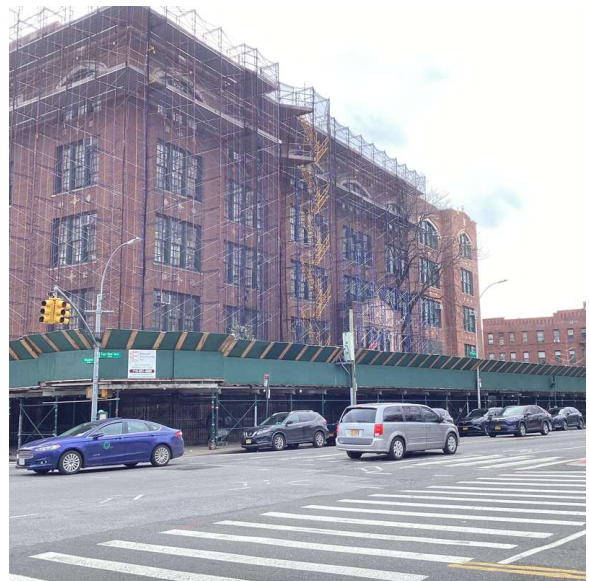
Corner of East New York Avenue and Rockaway Parkway - South View
