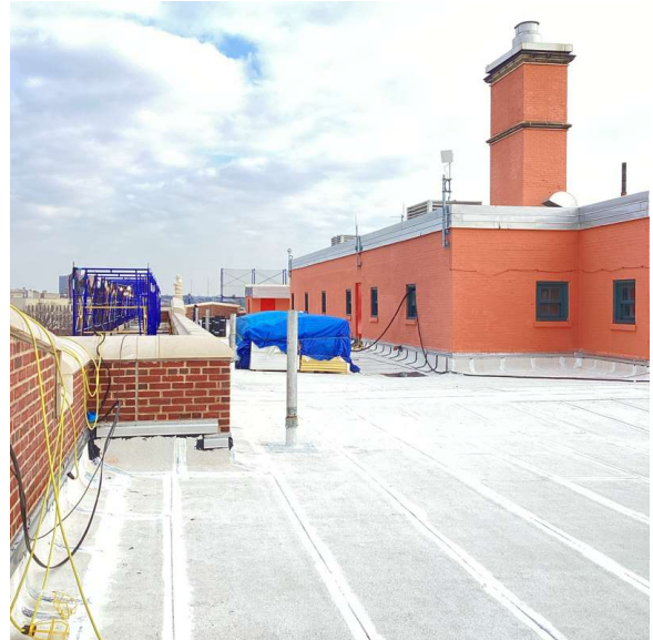
Roof 1 - Northeast View
